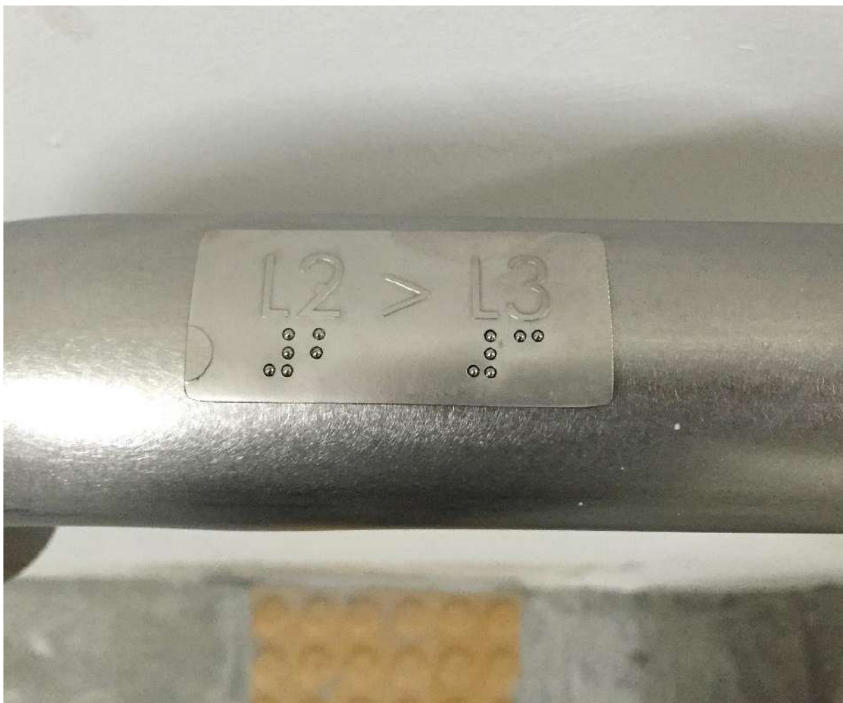
Image 11: Braille indicators at end of the handrails (Source: https://static.wixstatic.com/media/2f4db7_eab6b34aba264b0fab6143b2c80454fb~mv2_d_3264_2448_s_4_2.jpg )
