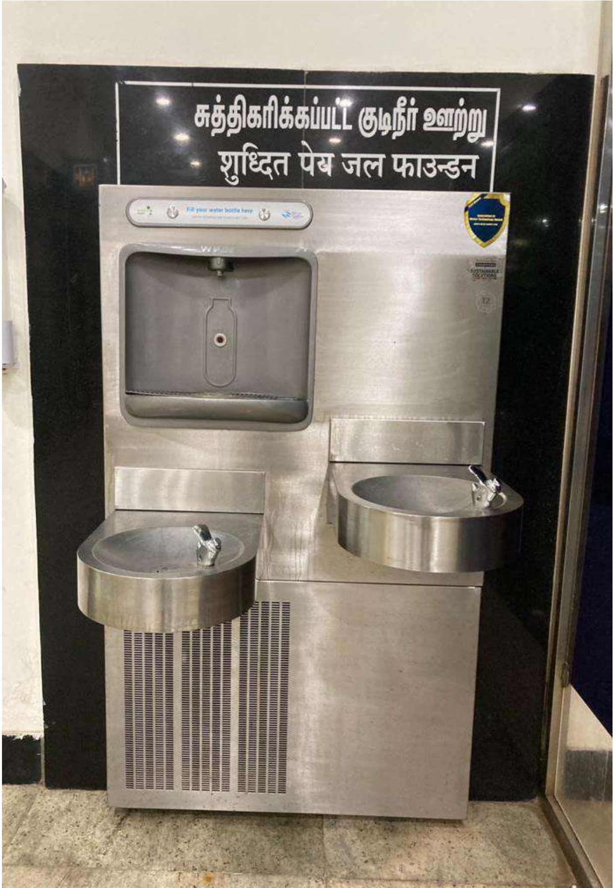
Image 16: Example of Drinking water facility with taps on two levels installed in Madurai Airport
